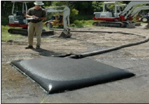
Plate 4-3 Silt Bag with water being pumped through
