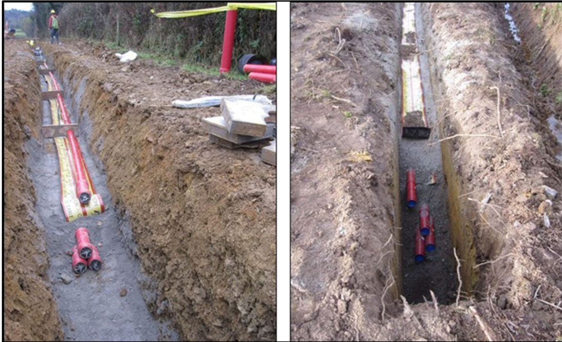
Plate 4-3 Standard Cable Trench View
