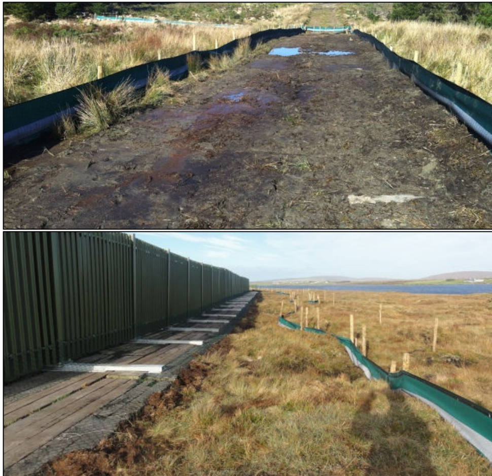
Plate 4-6 Silt Fence Details
