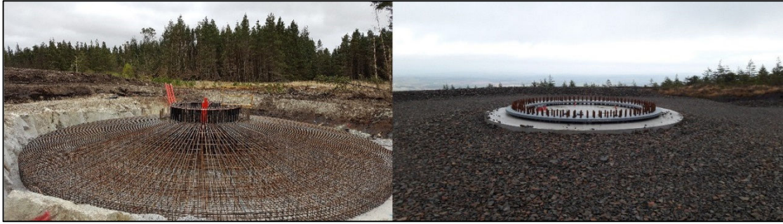
Plate 4-2 Turbine 'Anchor Cage' and finished turbine base
