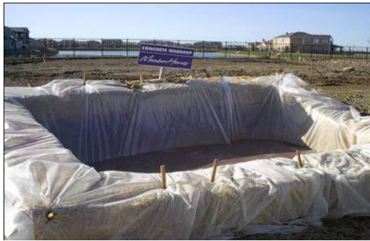
Plate 4-3 Concrete washout area
