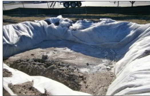
Plate 4-4 Concrete washout area
