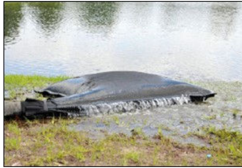
Plate 4-4 Silt bag under inspection
