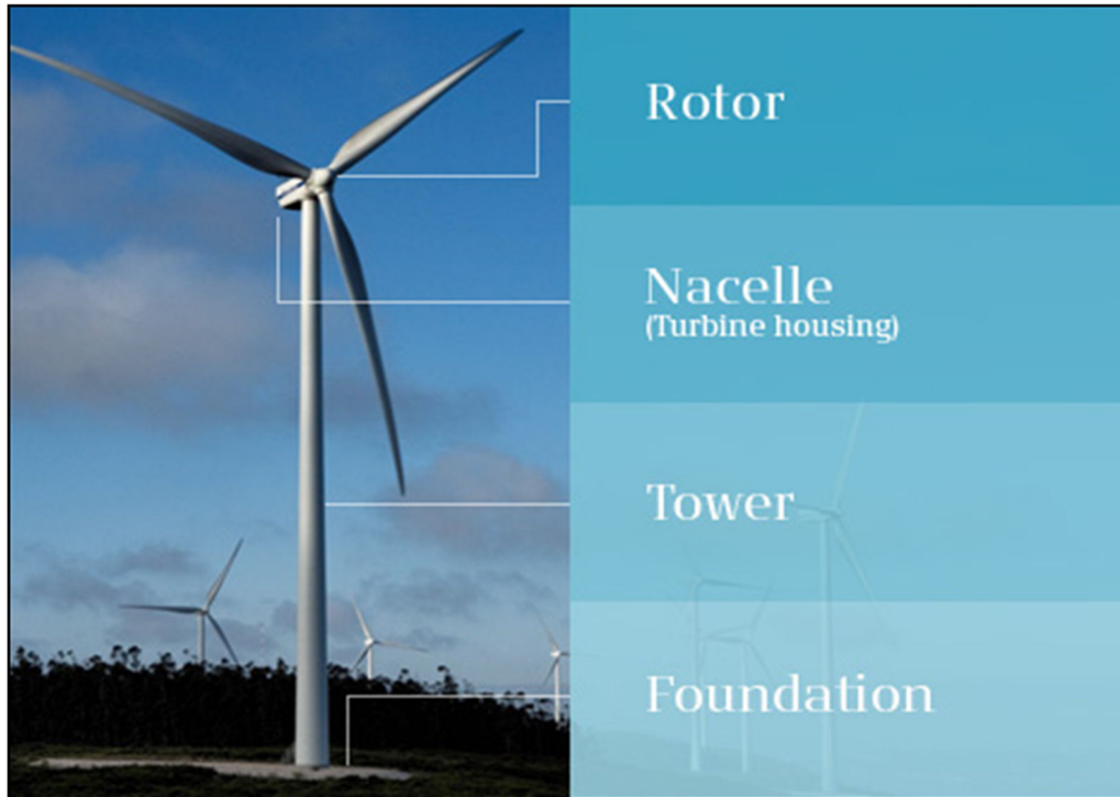
Plate 4-1 Wind turbine components
